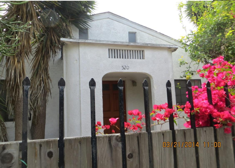
Front Existing Single Family Residence
