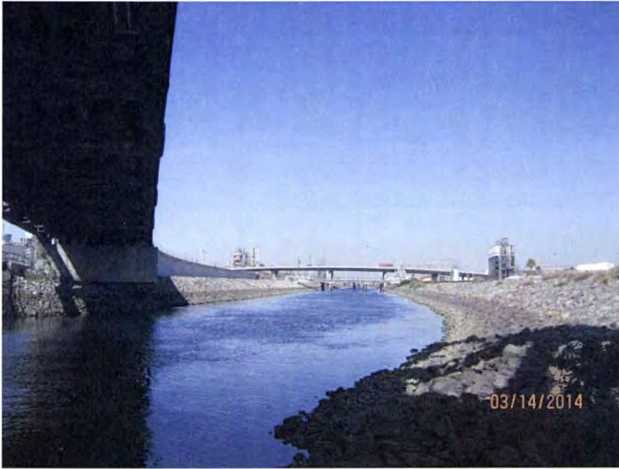
Photo 8. Photo showing the southern end of the channel where it opens to the Los Angeles Harbor. Banks are void of vegetation; however, several mollusks were observed attached to the rocks. Photo facing northwest.
