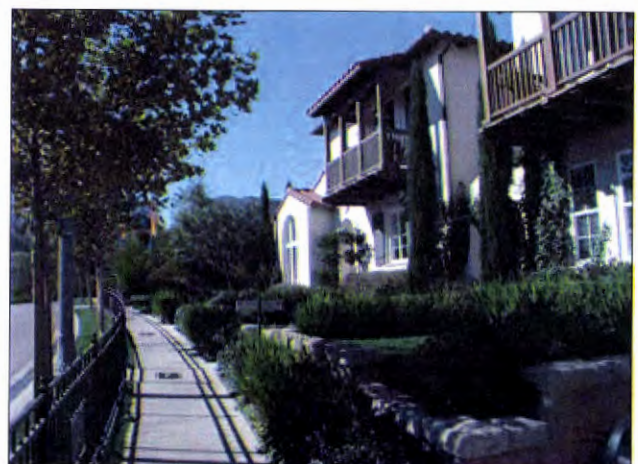
Illustrative Photo: balcony supported by cantilevered beams
