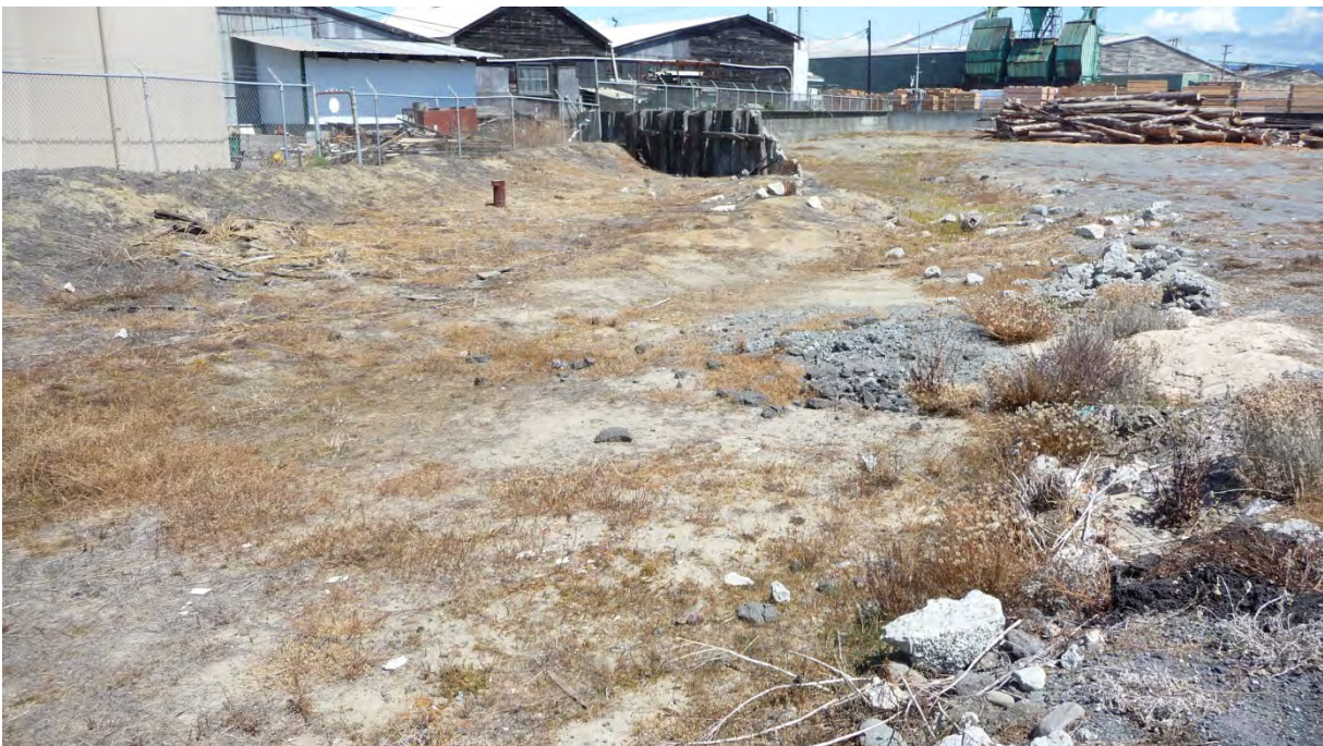
The eastern side of the Tank Farm 2 Containment Basin looking east towards the Tank Farm 1 Containment Basin. Tank Farm 2 was constructed with an earthen berm while Tank Farm 1 was constructed with a concrete berm.
