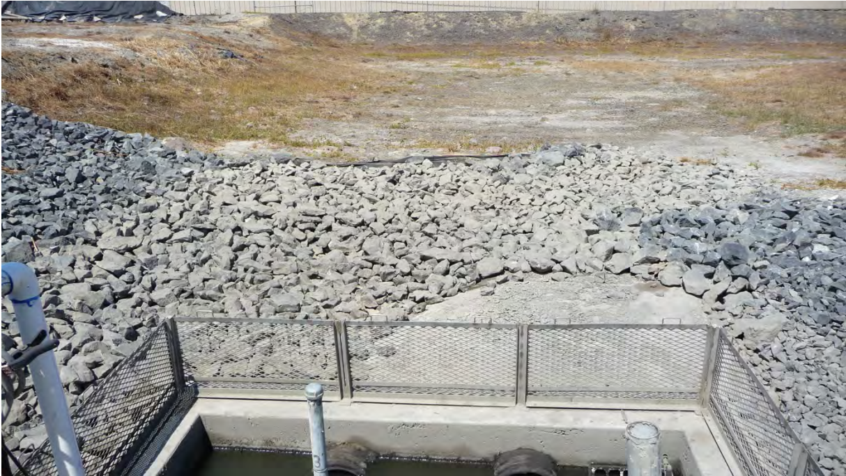
Settling pond at the western edge of the Tank Farm 2 Containment Basin. The rocks are used to trap sediment before the stormwater is pumped through the filters.
