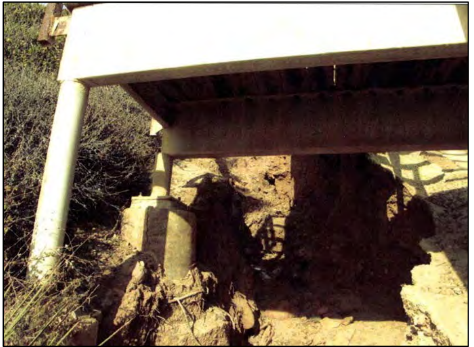
Exhibit 5 Stairway Erosion Photos MSB-NOID-0005-14
