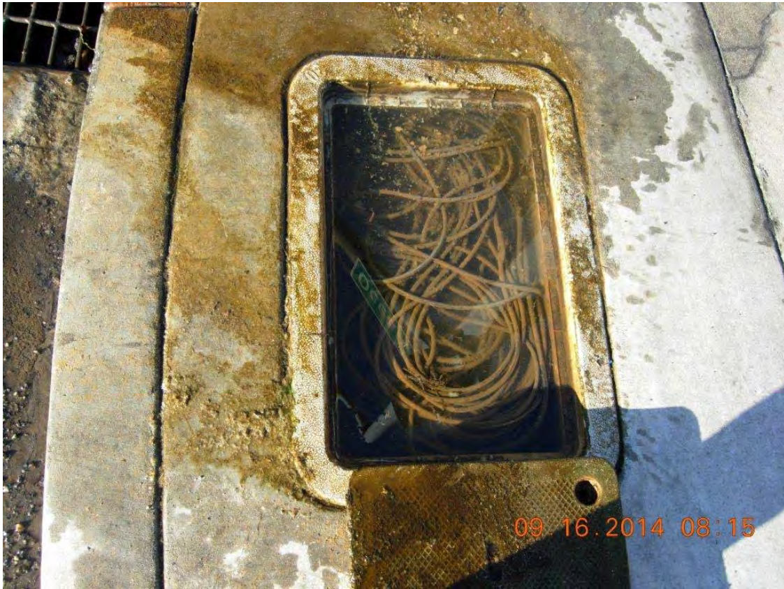
Photo 1: Flooded Electrical Box
