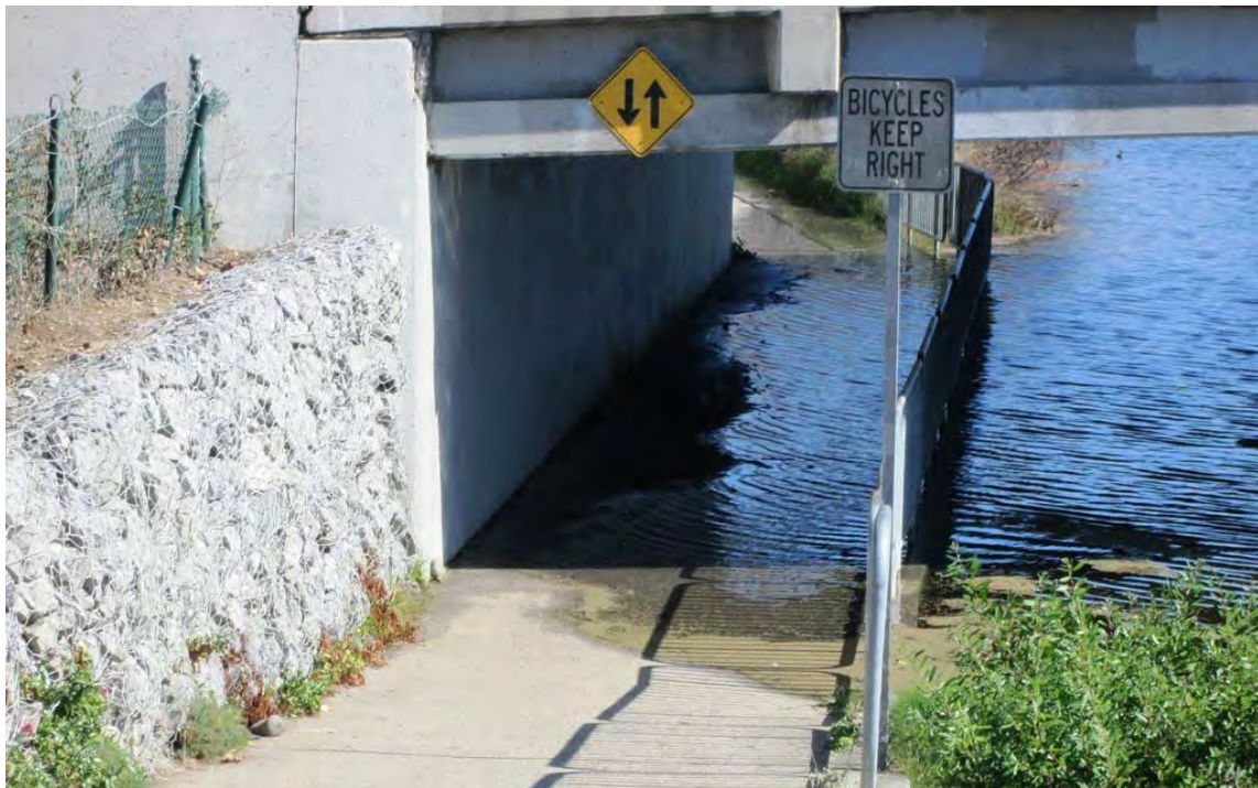
Photo 7: Flooded bike path at river
