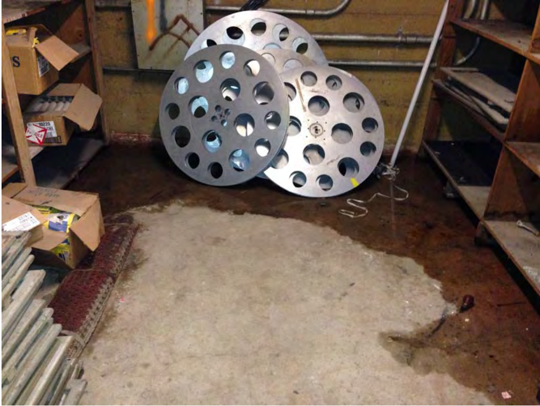
Photo 4: Del Mar Theater storage area flooding
