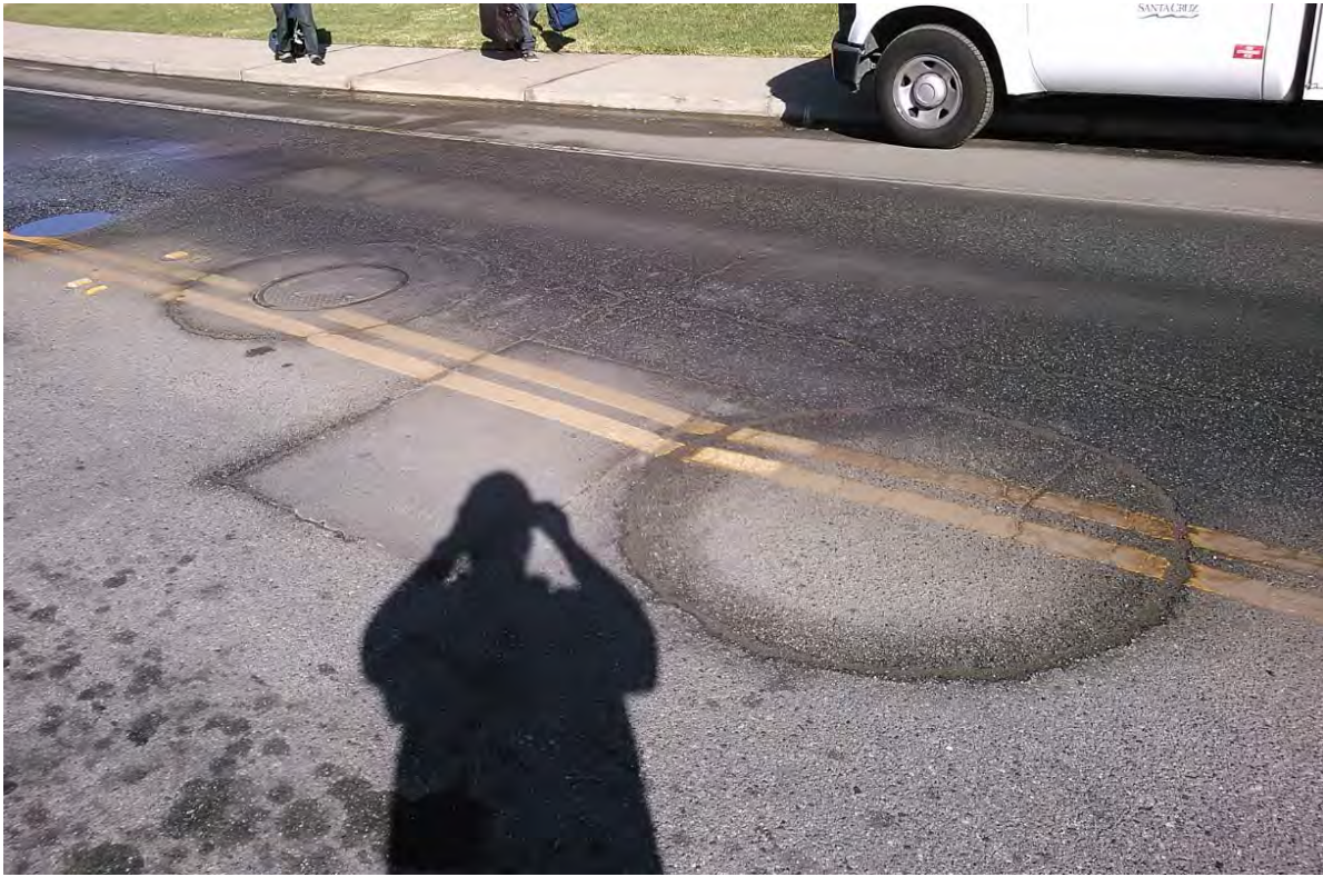
Photo 5: River water saturating Riverside Drive pavement and San Lorenzo River bikeway flooding, 2014. Photos by Revell Coastal.
