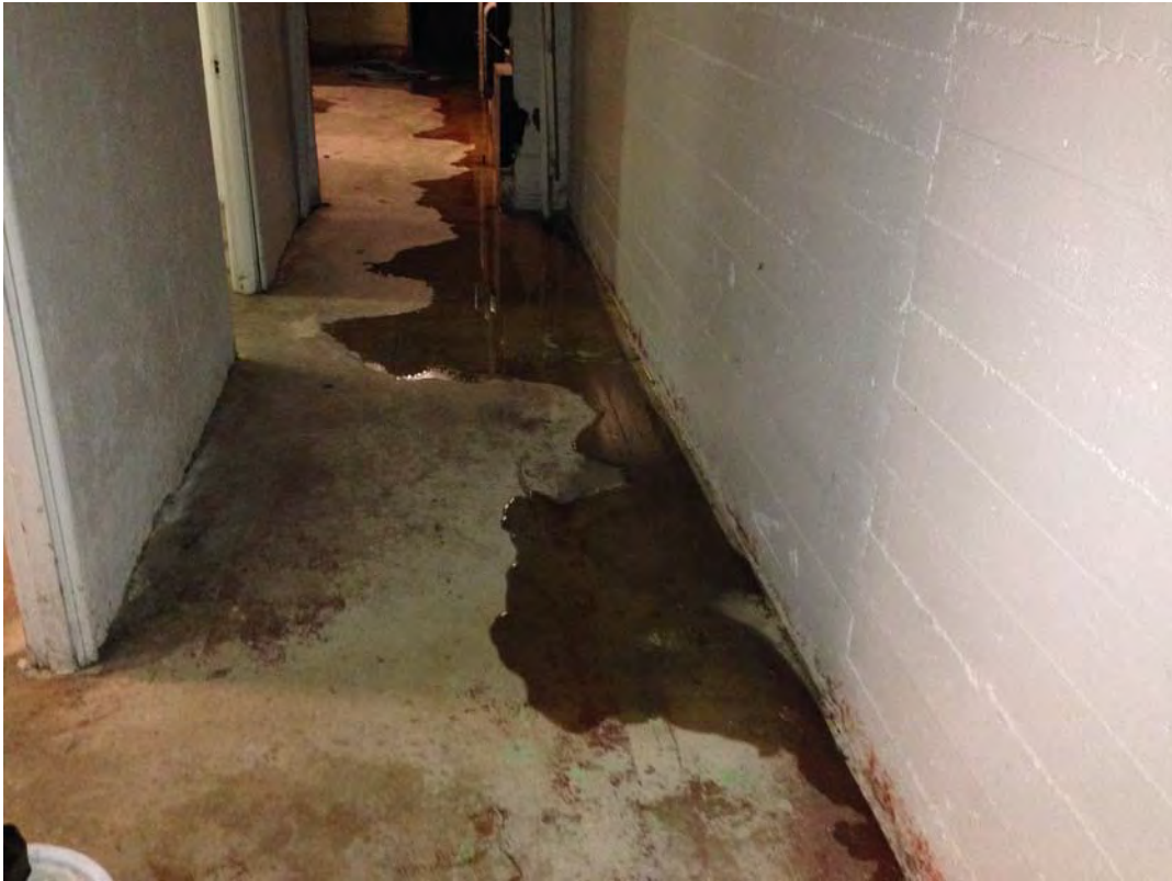
Photo 3: Del Mar Theater ground floor flooding
