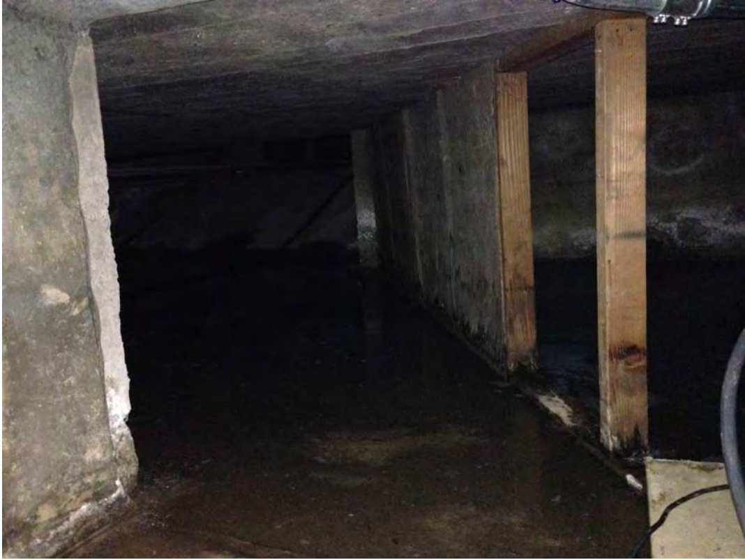
Photo 2: Del Mar Theater Basement flooding
