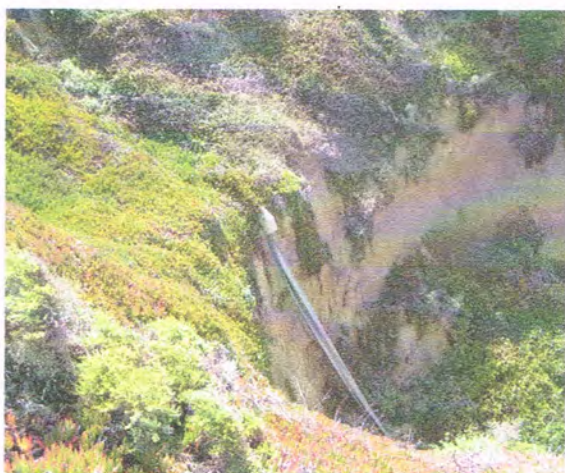
16" drain under Palmetto Ave empties into ravine. Note metal strip attached.
