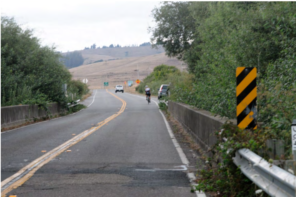
View of Bridge Shoulder with Cyclist, Facing North
