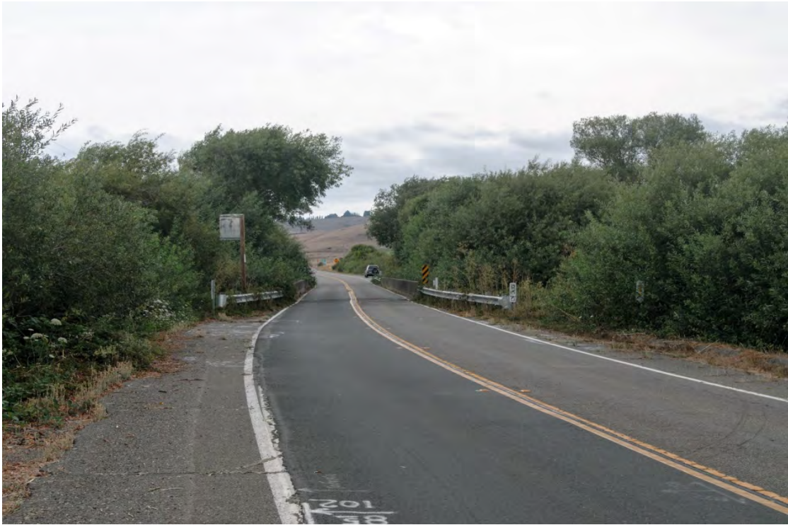
View of Bridge and Bridge Shoulder, Facing North
