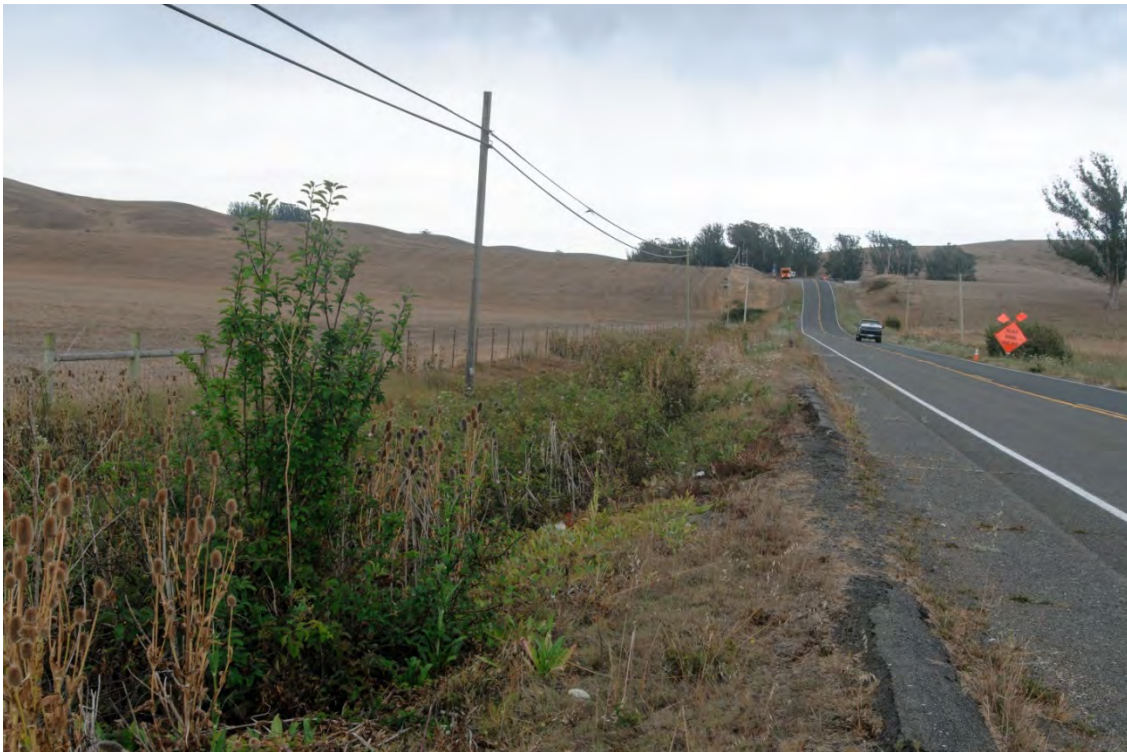
View of Bridge Shoulder and Roadway Embankment, Facing South
