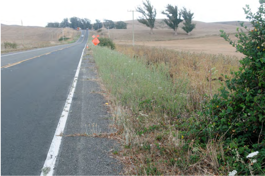
View of Roadway Shoulder and Embankment, Facing South, Just Beyond the Bridge
