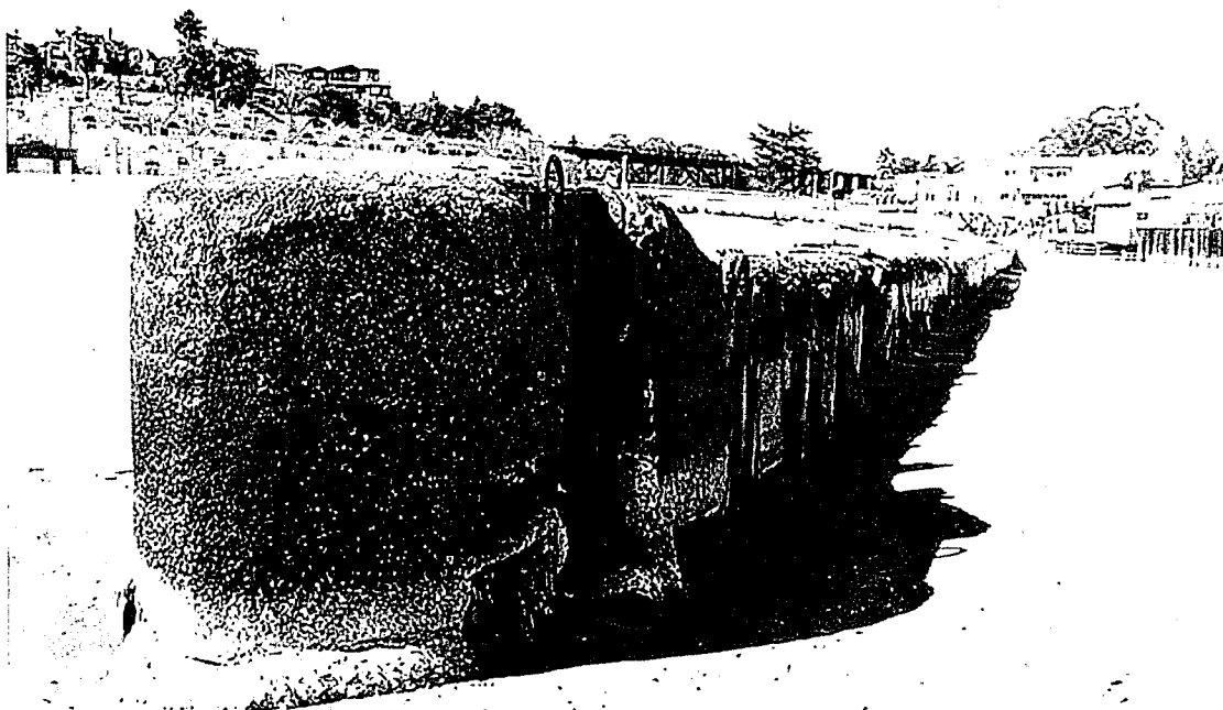
Photo 1: Note cement bulkhead of flume extending into ocean mid-beach.
