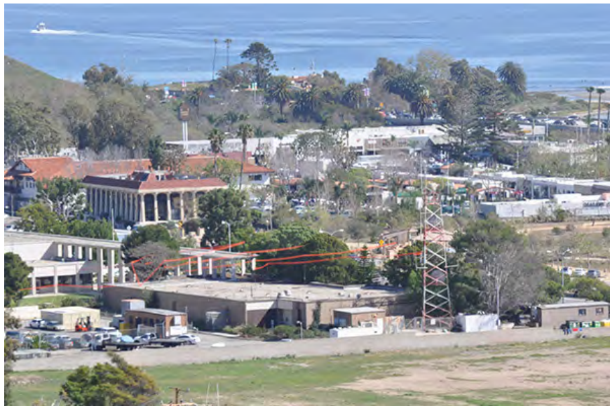
Zoomed-in View of the Project Site with Story Poles from Malibu Knolls. There are no scenic or visual impacts due to the height of the building.
