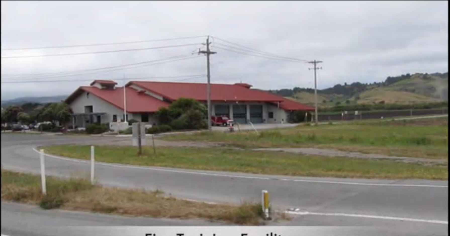
Fire Training Facility Traveling North on Highway 1
