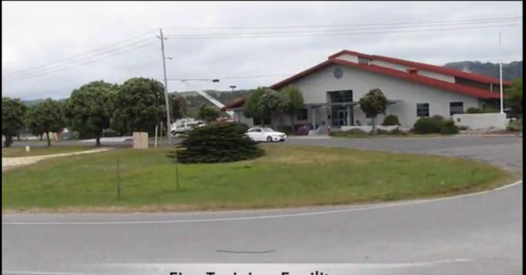
Fire Training Facility Traveling North on Highway 1
