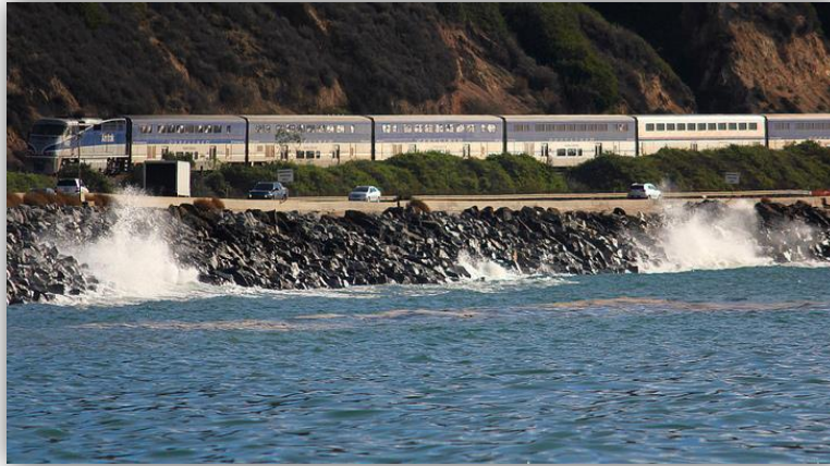
Figure 7. Photo of infrastructure at risk near Rincon Beach, Ventura, CA, during the King Tide in December 2012. (Photo courtesy of David Powdrell, California King Tides Initiative)
