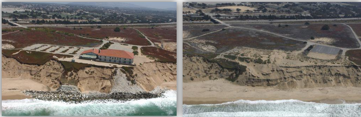
Figure 15. Photo depicting passive erosion. (Left) Passive erosion in front of a revetment at Fort Ord, illustrating the loss of beach where the development prevents the shoreline from migrating landward. The beach continues to migrate inland on either side of the revetment. (Right) Recovery of the beach following removal of the revetment and blufftop structure. (Source: California Coastal Records Project ).
