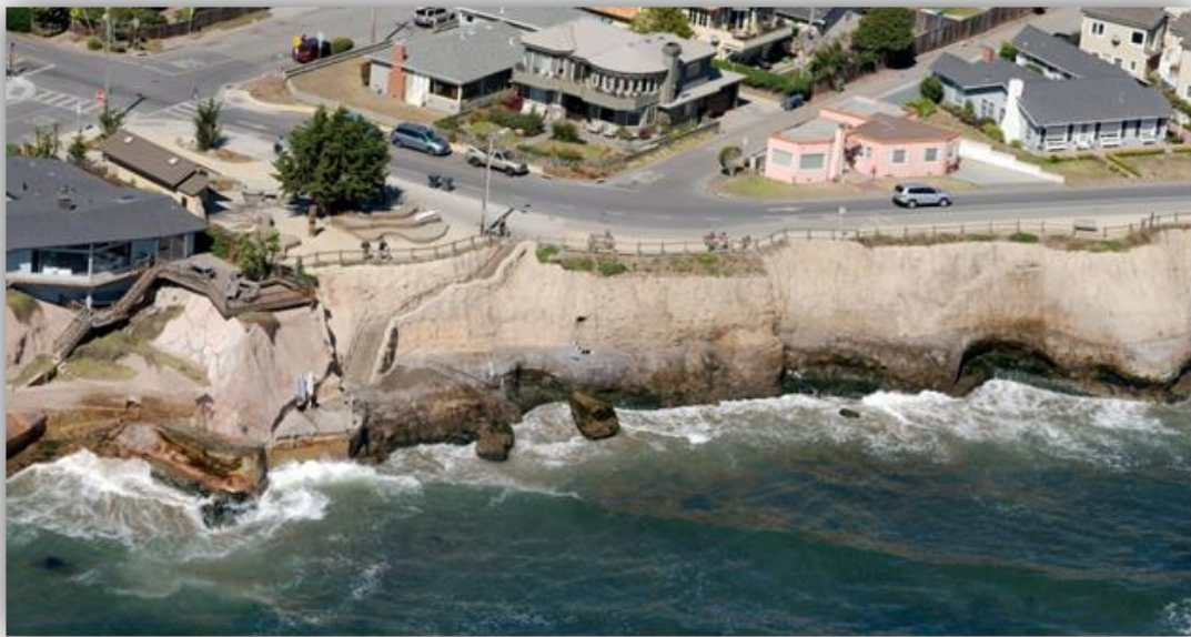
Figure 25. Photo depicting protection of visual resources and public access. A seawall visually blends in with the natural bluff while surfing access is also provided at Pleasure Point, Santa Cruz (2013). (Source: California Coastal Records Project )
