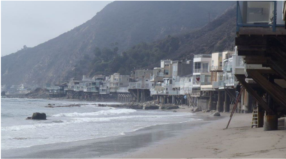
Development in Malibu abuts the sea and is particularly vulnerable to beach erosion. Photo Credit: Lesley Ewing
