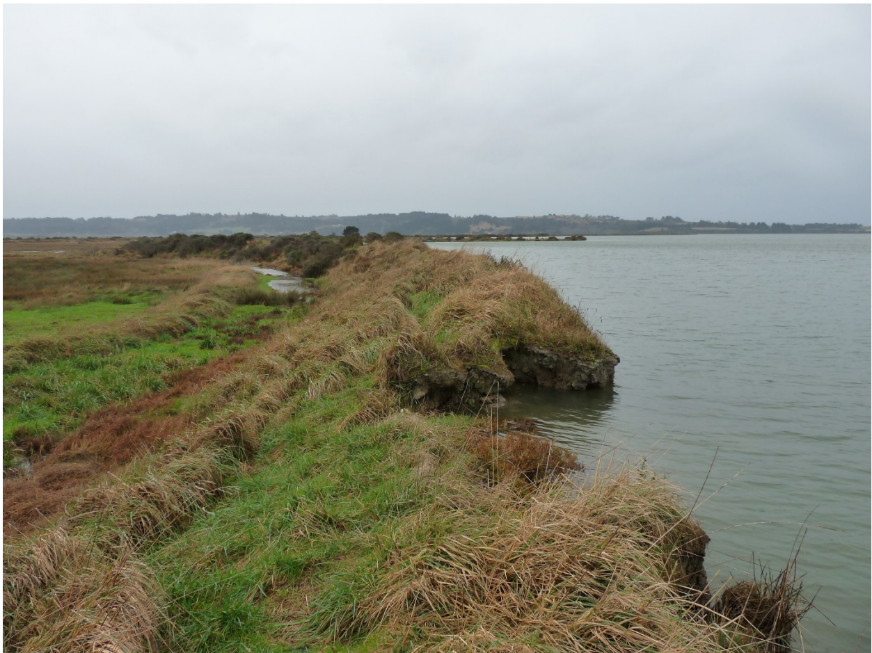
Figure 9. Eroded and low elevation diked shorelines on the Humboldt Bay National Wildlife Refuge in South Bay are vulnerable to breaching during king tides and/or storm surges.
