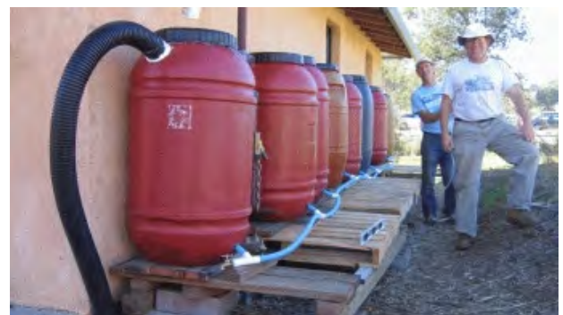
Daisy-chained system Courtesy of Acterra
