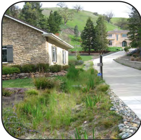
Large Residential Rain Garden
