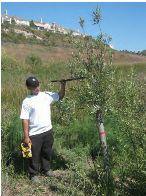
Installing willows at Upper Newport Bay
