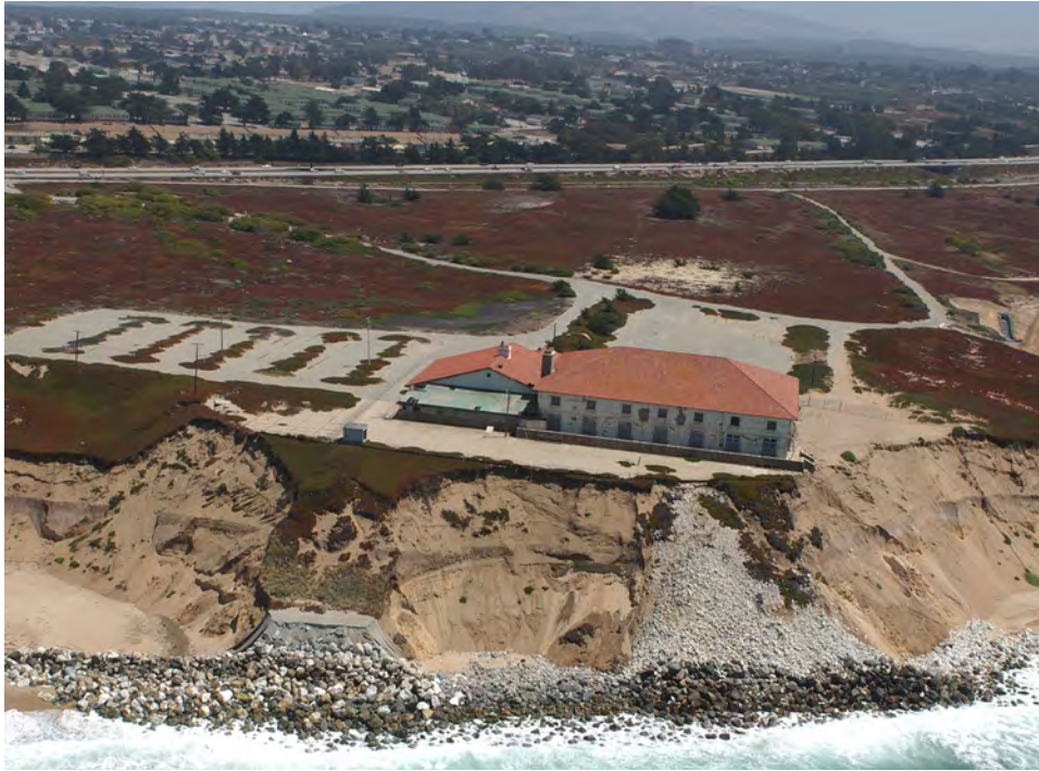
Stilwell Hall, Fort Ord. Facing bluff erosion, this World War II era building was demolished in 2003. Copyright (C) 2003 Kenneth & Gabrielle Adelman, California Coastal Records Project
