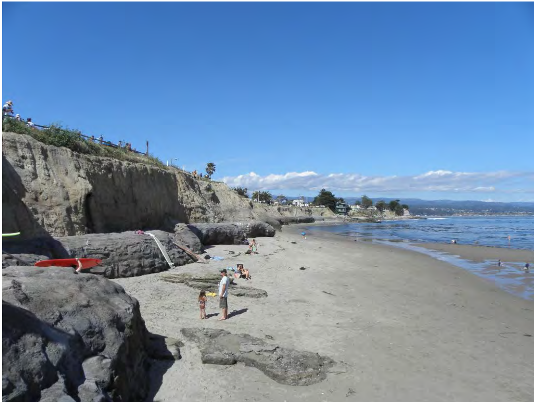
Figure 2: Photo of Seawall at Pleasure Point. Designed and built to blend with natural bluff conditions.
