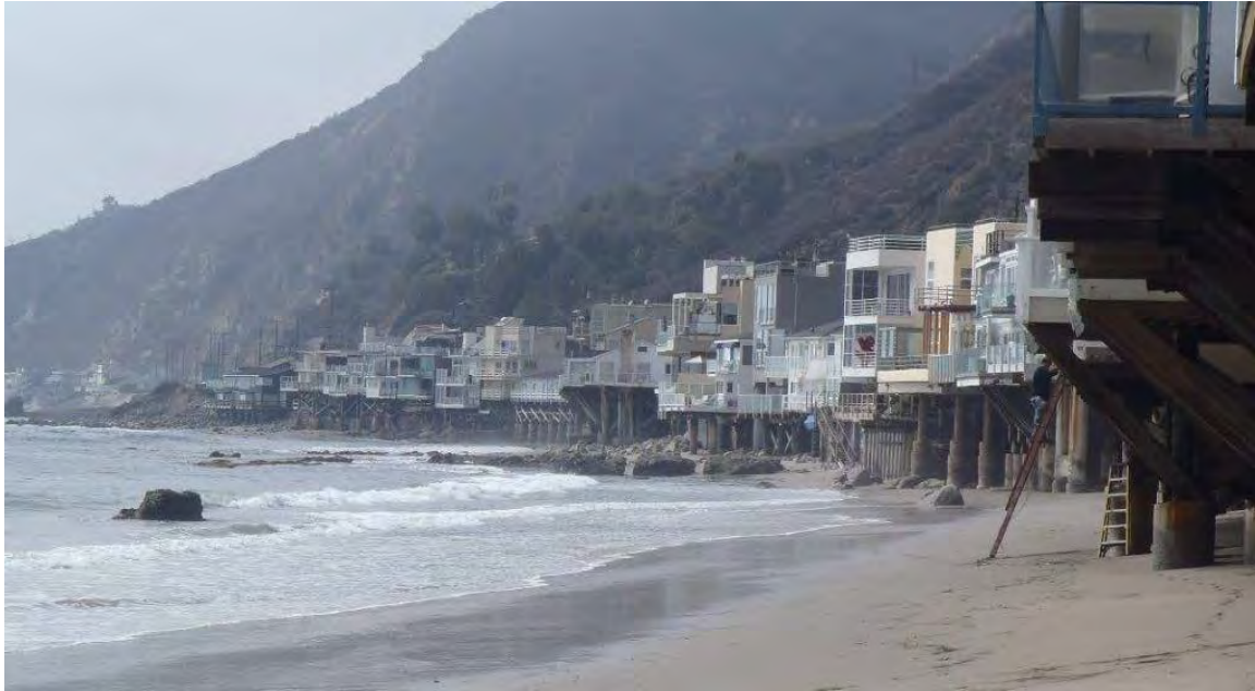
Development on Broad Beach in Malibu abuts the sea and is particularly vulnerable to beach erosion. Photo Credit: Lesley Ewing
