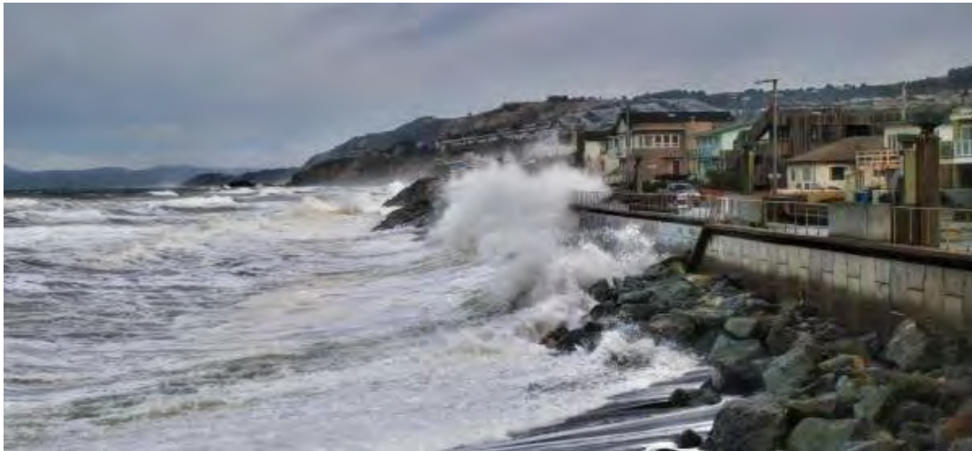
Development along Pacifica is battered by the surf during a King High Tide; the beach is non-existent. Photo Credit: Jack Sutton
