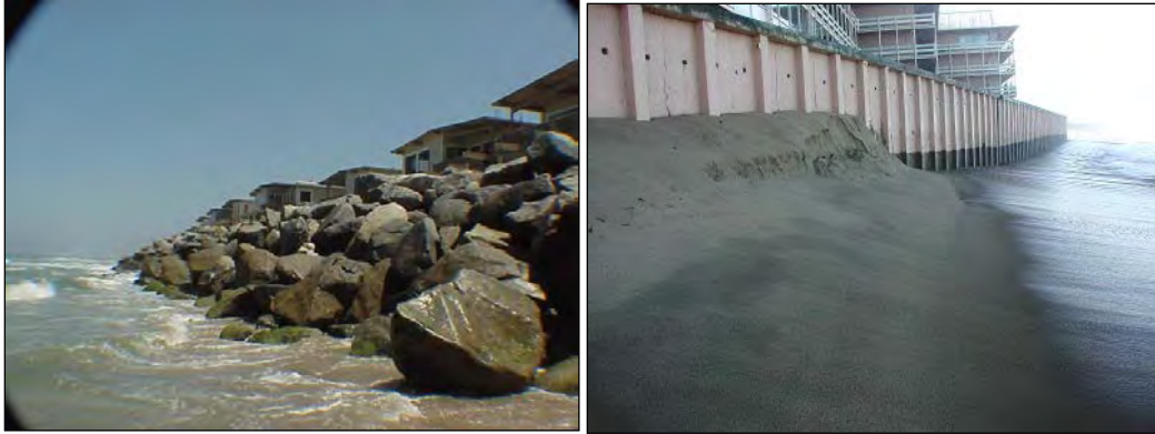
Figure 3: Shoreline Armoring Structures: a rock revetment in San Clemente, CA and a seawall in Monterey, CA. Source: Surfrider Foundation
