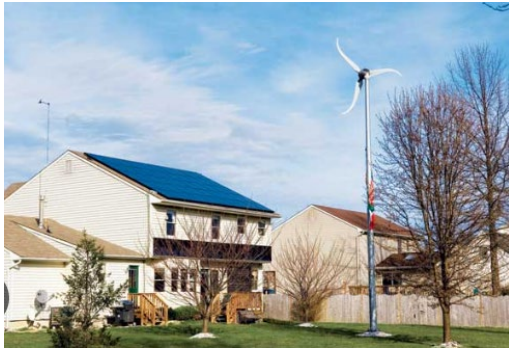
Roof-mounted solar and ground-mounted wind
