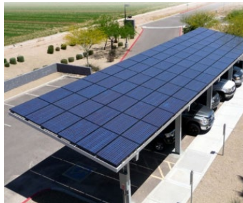
Carport roof-mounted solar
