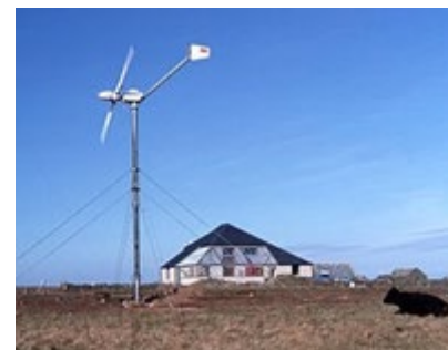
Ground-mounted wind turbine
