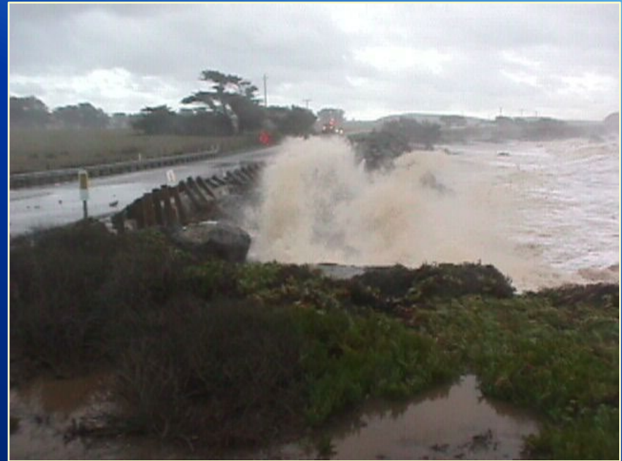
Photo: Wave impact, with erosion and overtopping of 17-Mile Drive in Pebble Beach.
