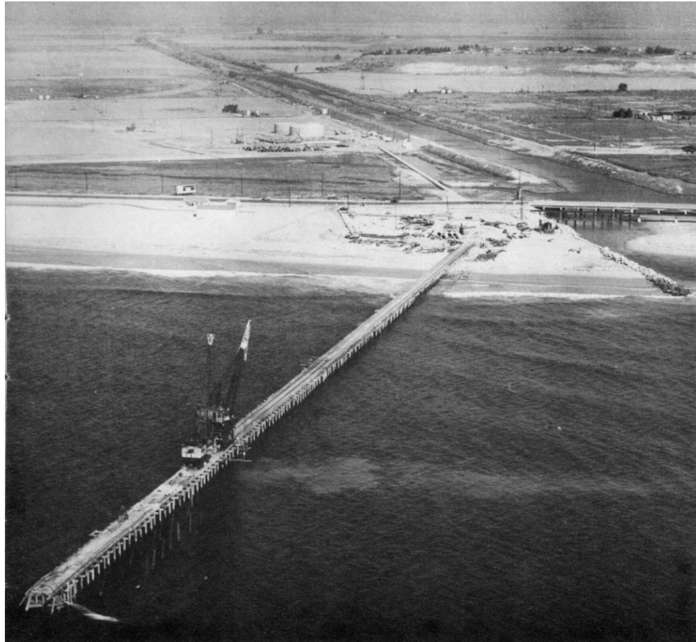
Figure 3.3 Typical trestle construction
