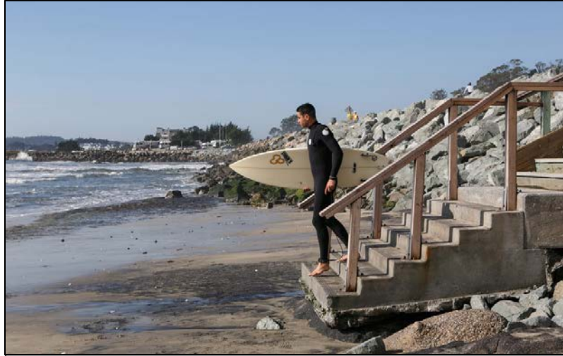
A surfer uses the repaired beach access stairs at Surfers Beach in Half Moon Bay.
