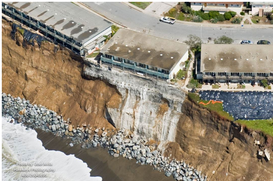
Bluff retreat in Pacifica ultimately led to the demolition of these apartments.
