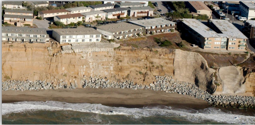
Figure 6. Photo of Esplanade Apartments threatened by cliff erosion in 2013 in Pacifica, CA. (Source: California Coastal Records Project )
