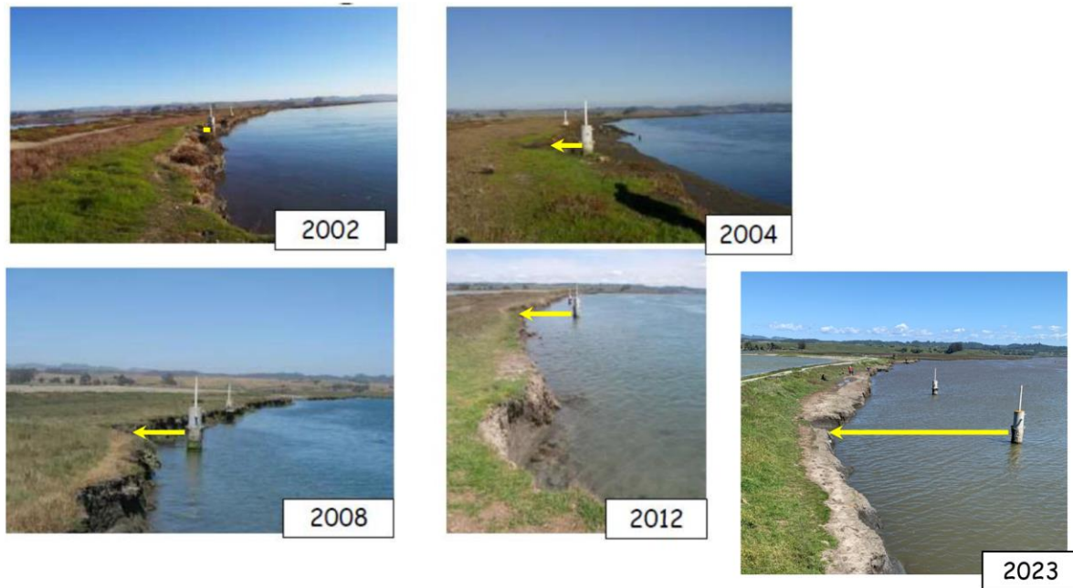
Figure B-3. Photo series documenting rapid bank and wetland erosion in Elkhorn Slough (adapted from California Department of Fish and Wildlife, 2021 with additional photo from B. Ammen, 2023)
