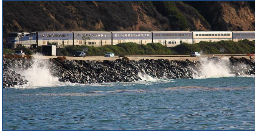
Figure 9. Photo of infrastructure at risk near Rincon Beach, Ventura, CA, during the King Tide in December 2012. (Photo courtesy of David Powdrell, California King Tides Initiative)
