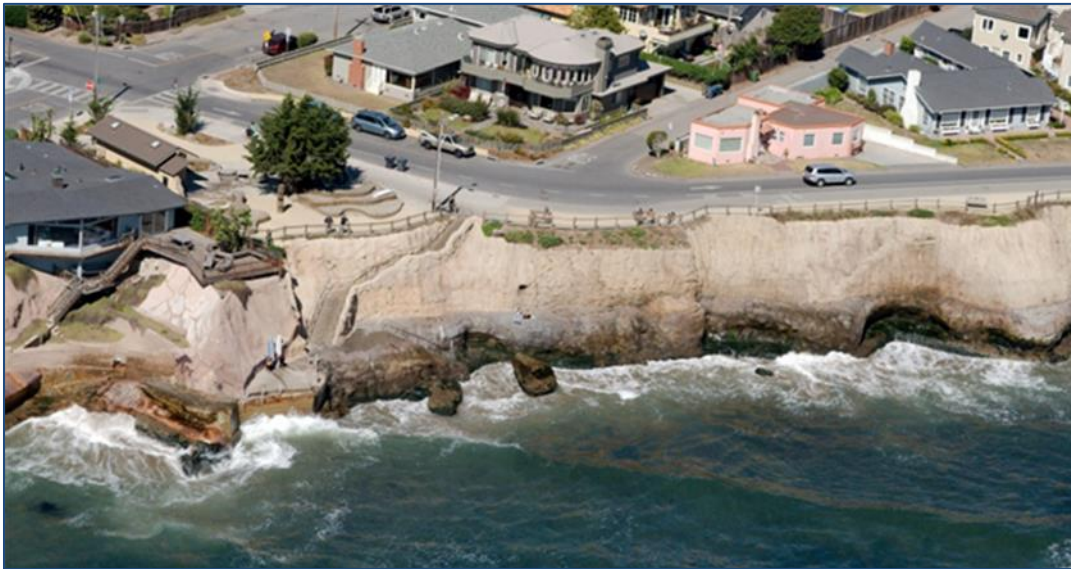
Figure 28. Photo depicting protection of visual resources and public access. A seawall visually blends in with the natural bluff while surfing access is also provided at Pleasure Point, Santa Cruz (2013). (Source: California Coastal Records Project )
