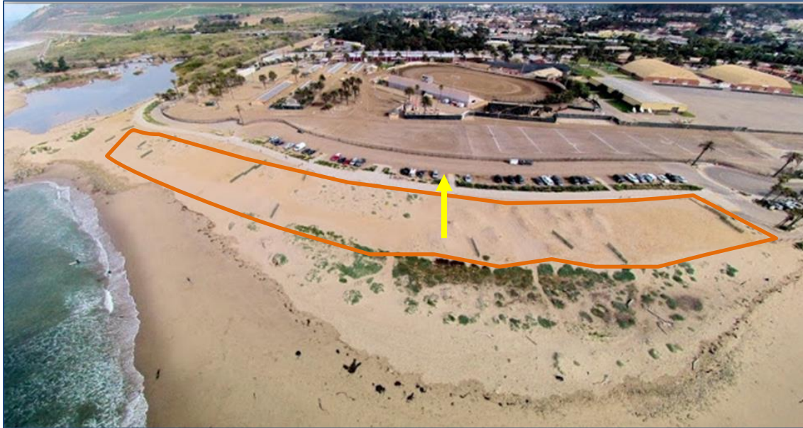
Figure 19. Photo depicting “managed retreat” and restoration. Surfers' Point Managed Shoreline Retreat project in which the parking lot was moved back and beach area was restored. (Aerial composite by Rick Wilborne (February 28, 2013); photo courtesy of Surfrider Foundation)
