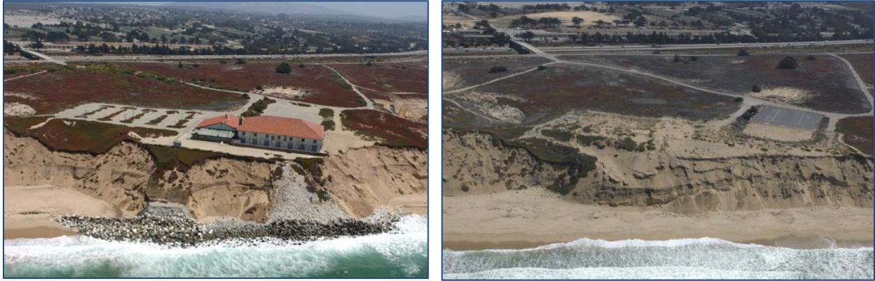
Figure 18. Photo depicting passive erosion. (Left) Passive erosion in front of a revetment at Fort Ord, illustrating the loss of beach where the development prevents the shoreline from migrating landward. The beach continues to migrate inland on either side of the revetment. (Right) Recovery of the beach following removal of the revetment and blufftop structure. (Source: California Coastal Records Project ).
