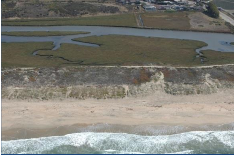
Figure 27. Photo depicting habitat protection at Salinas River State Beach. Dunes are roped off to protect Snowy Plover nesting habitat. (Source: California Coastal Records Project )
