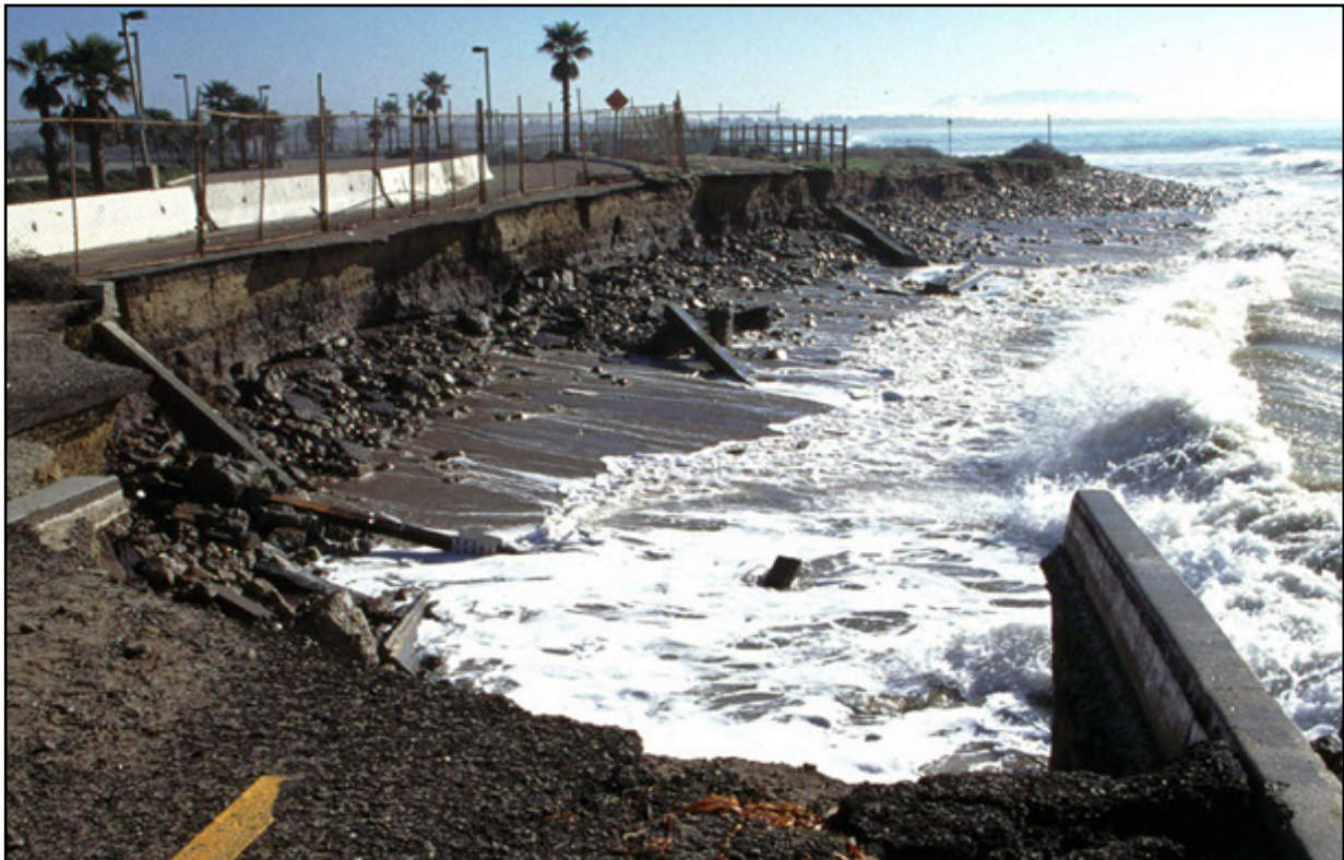
Figure E-6. Photo of eroded bike path and fill after storms in 1997 (Paul Jenkin, Surfrider Foundation).
