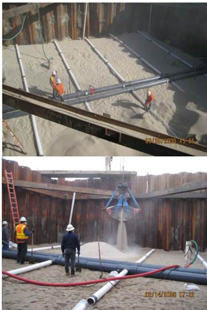
Fig. 9. Construction of the City of Long Beach, California seabed gallery system. This gallery required the use of sheet-piling and temporary dewatering to install the gravel and screen system.
