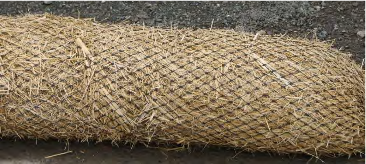
A fiber roll (straw wattle) with plastic netting, used for sediment control during construction in Trinidad, California. (Photo: Vanessa Metz, California Coastal Commission)
