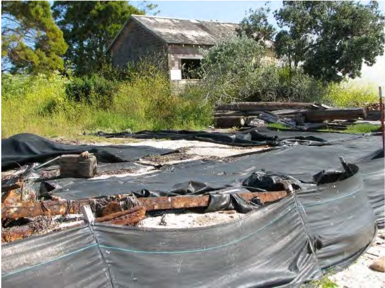
A degraded geotextile silt fence in Eureka, California. (Photo: Vanessa Metz, California Coastal Commission)
