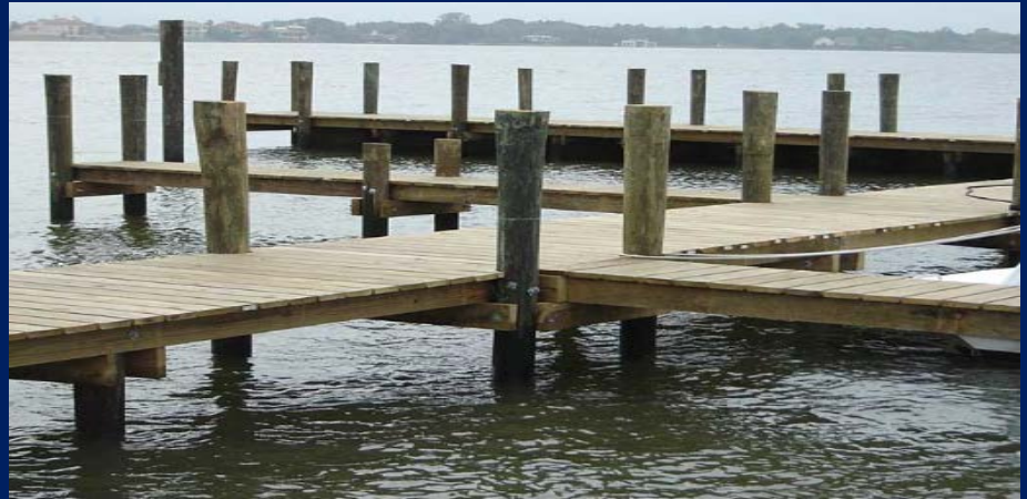
Treated wood decking, piles and structural framework
