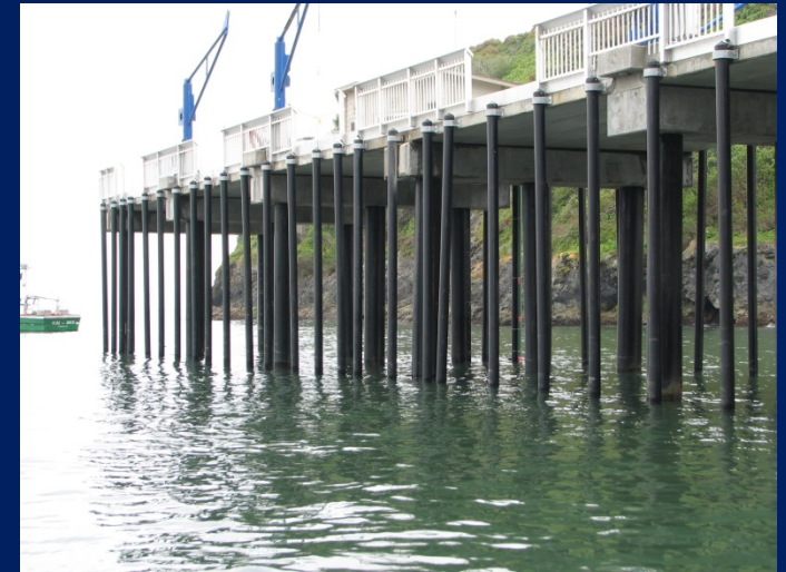
Plastic-wrapped concrete piles
