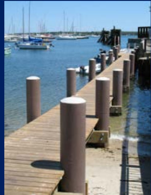
Fiberglass polymer piles
