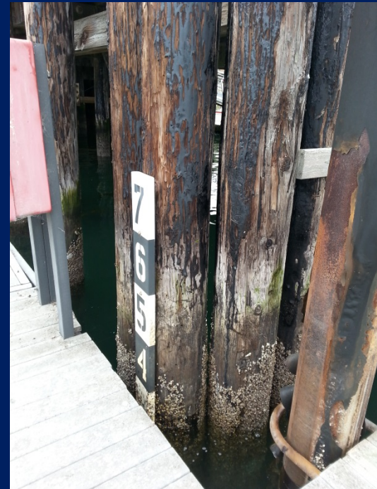
Creosote treated piles in center
