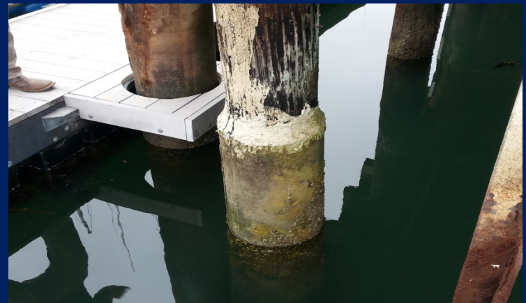
Epoxy-filled fiberglass jacket
