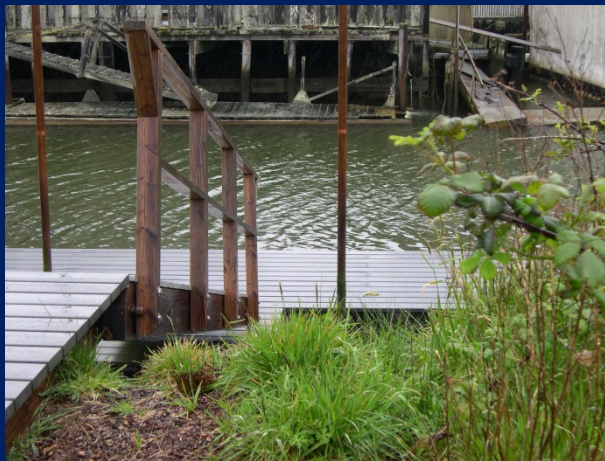
Composite decking on redwood frame
