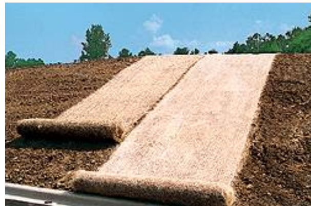
Temporary Rolled Erosion Control Product (RECP)
