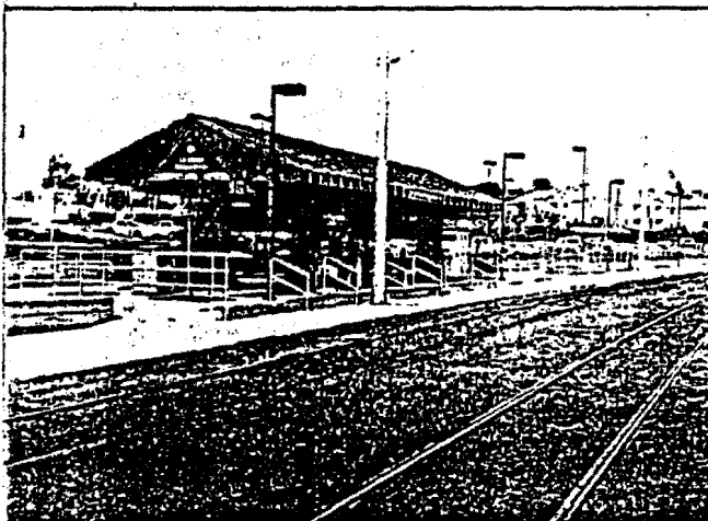
Standard station shelter with paved trackway.
