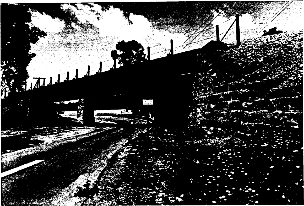
PHOTO 23: Los Patos Way Railroad Bridge
