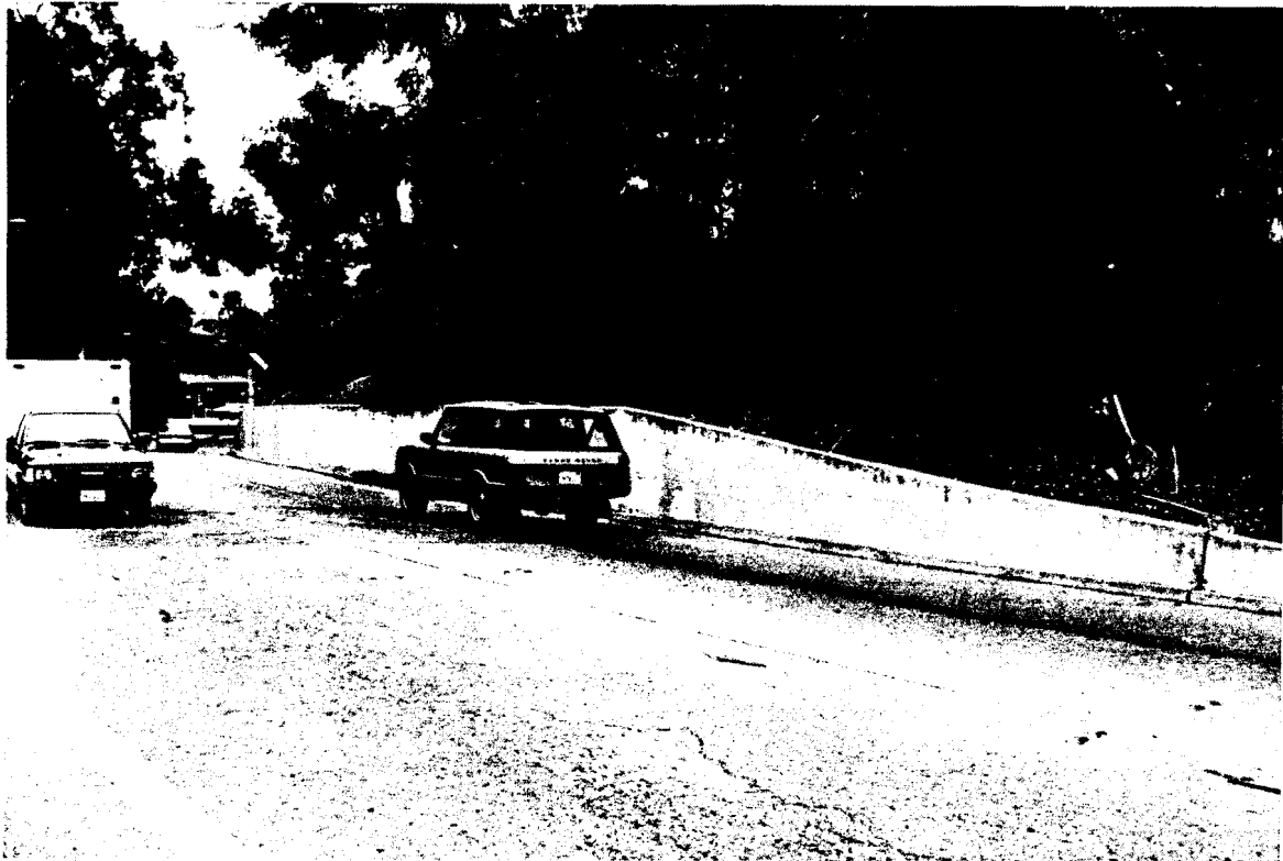
PHOTO 1: Retaining Wall at Hot Springs Road/Cabrillo Boulevard Interchange
