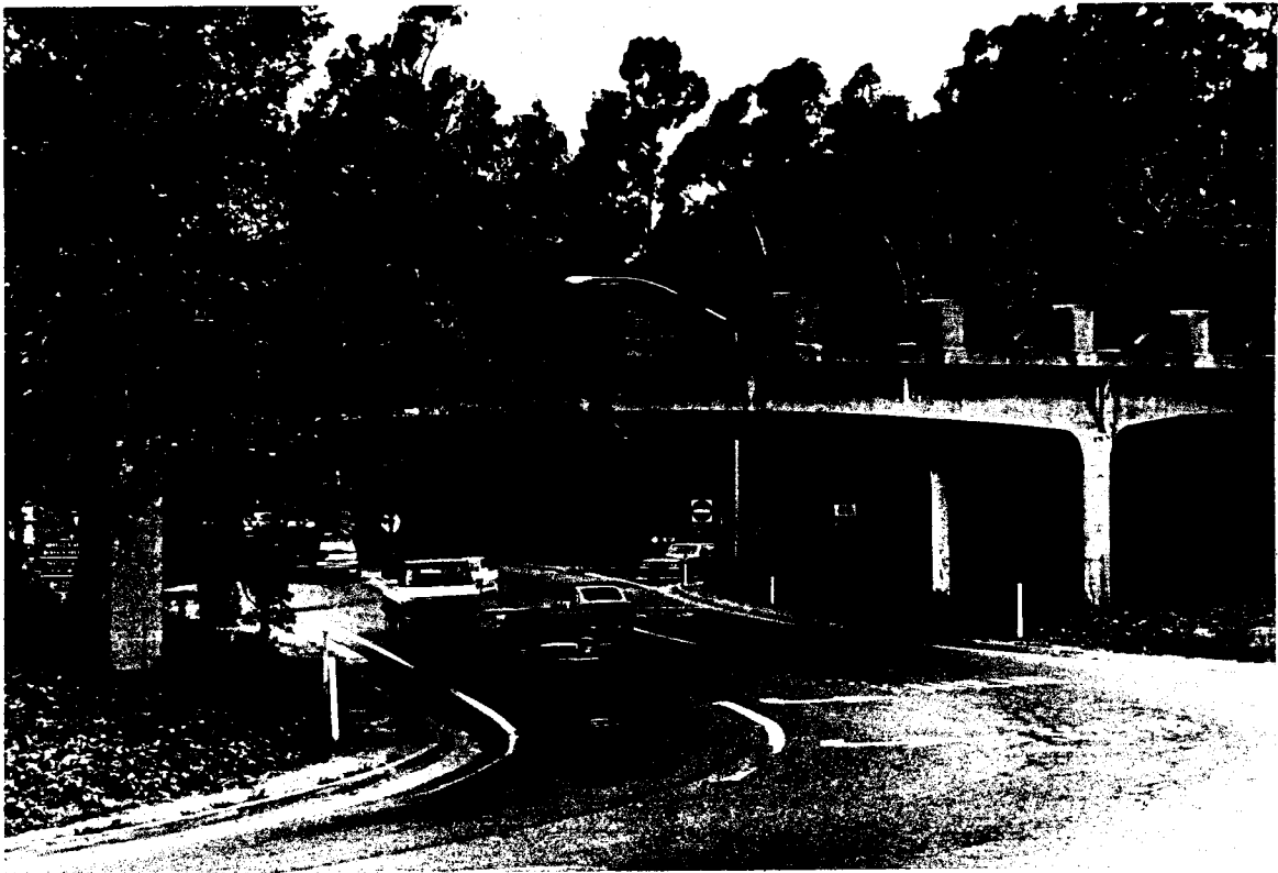
PHOTO 7: Hot Springs Road/Cabrillo Blvd. Interchange landscaping: Looking south from northbound on-ramp
