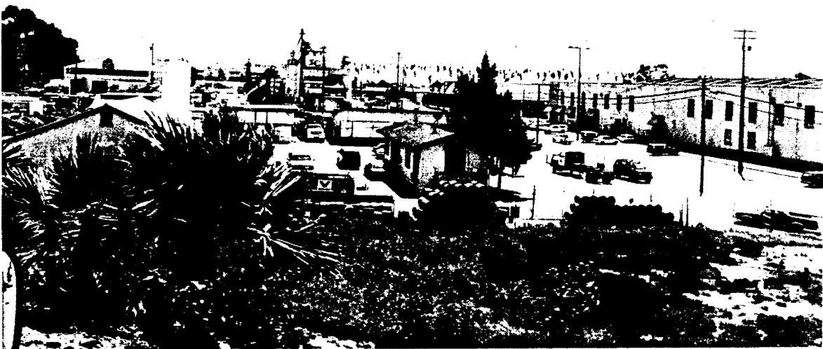
PHOTO 11: Industrial area looking toward beach
