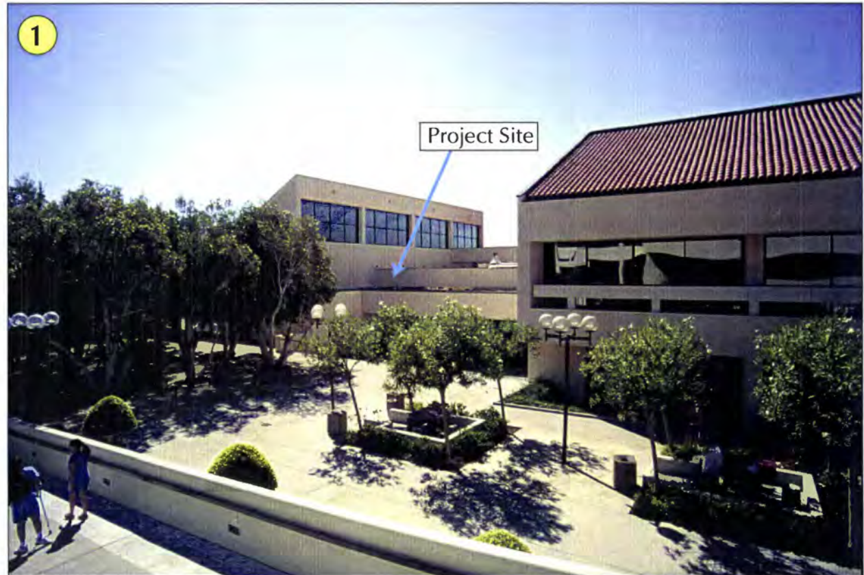
View of Proposed Tyler Campus Center Roof Expansion Site Looking Southeast.
