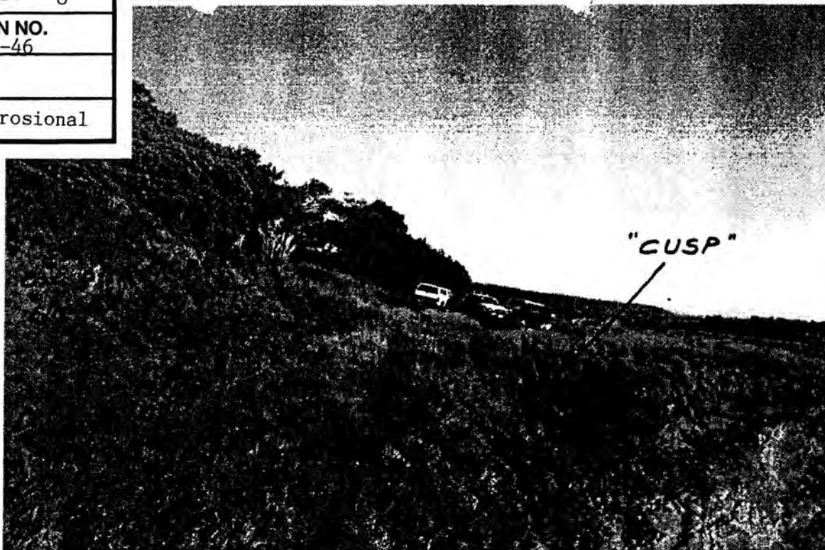
Photo 6: Erosional "cusp" in marine terrace, as seen from just north of the cusp, at the crown of the sea cliffs. The proposed driveway alignment skirts this feature. The old railroad embankment is at left. Note trail, which directs runoff to this location.
