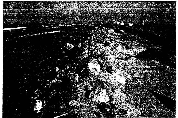
Western Seawall, east section view to west. Note scatter of large rocks.
