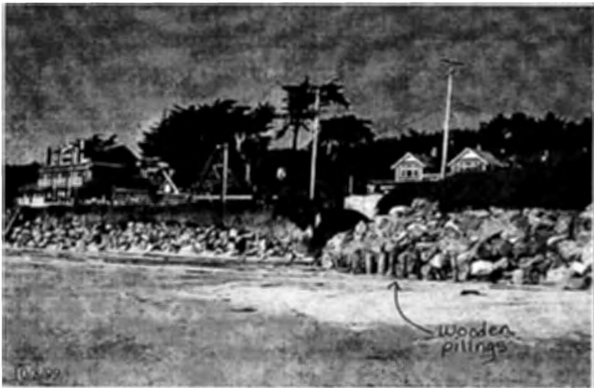
Photo 4: Northern portion of revetment (near river outlet)
