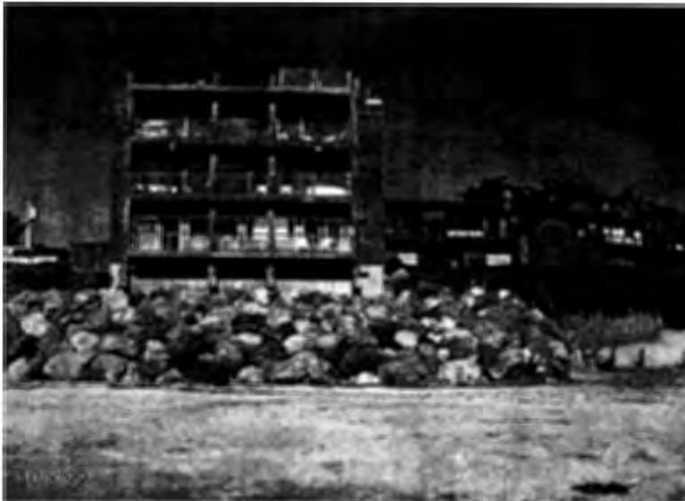
Photo 2: Apartment Building (looking east) with townhouses behind
