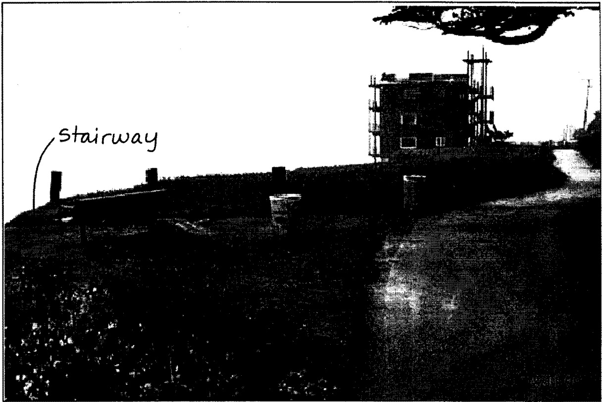
Photo 5: View of apartment building (looking northwest)
