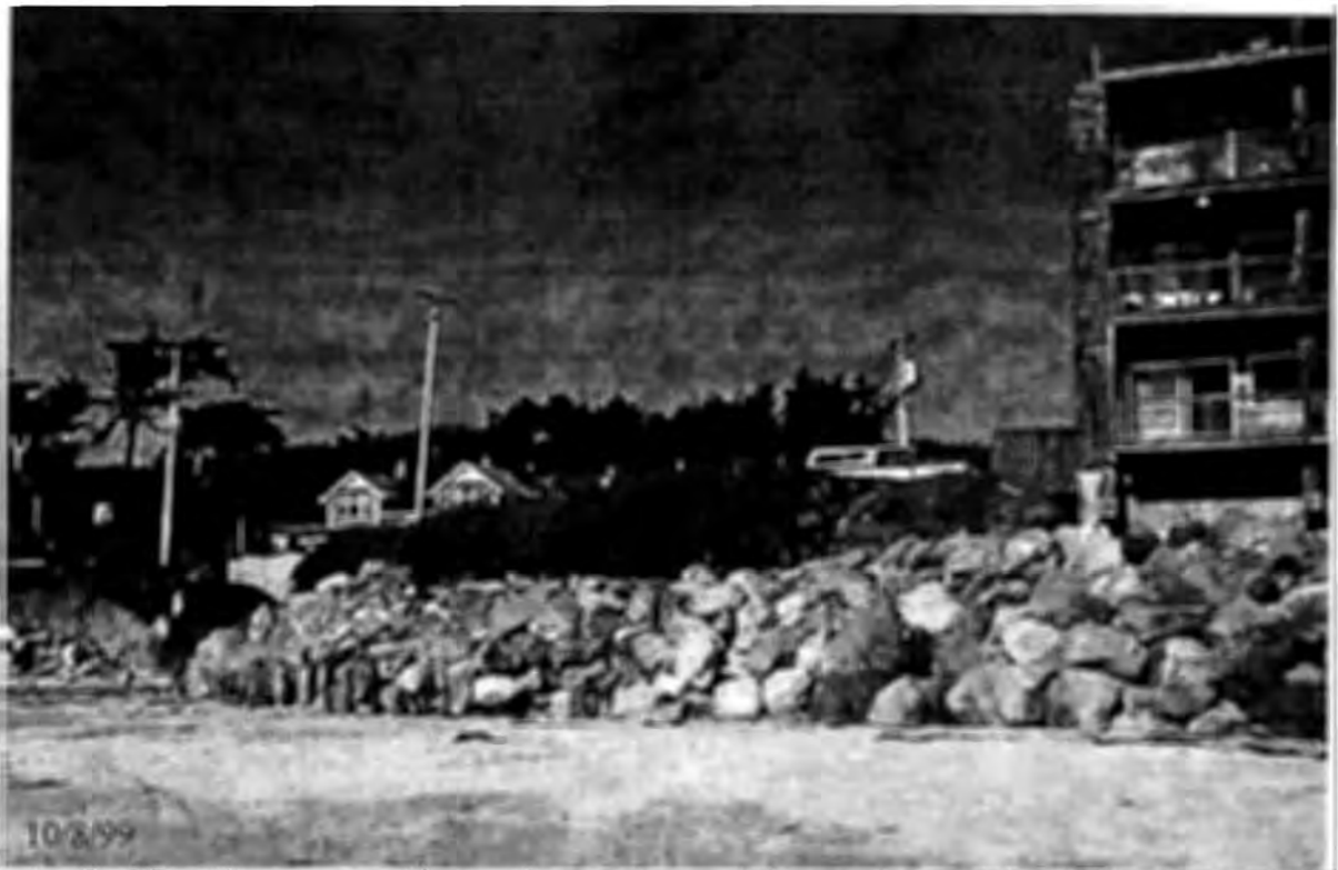
Photo 3: Northern portion of revetment (apartment building on right)
