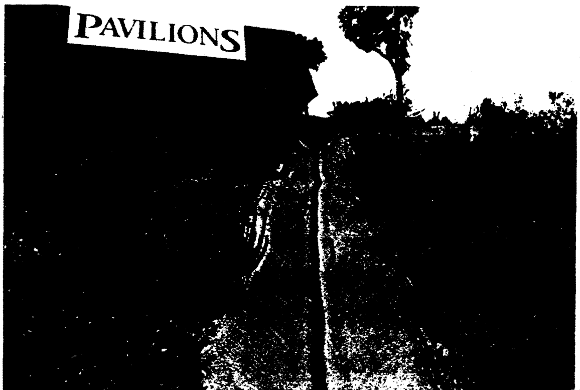
Photograph C - View of V-ditch which currently discharges onto site.
