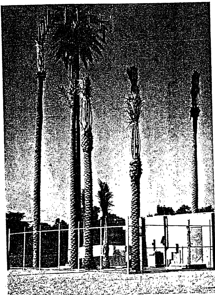
Monopole disguised as a palm tree.
