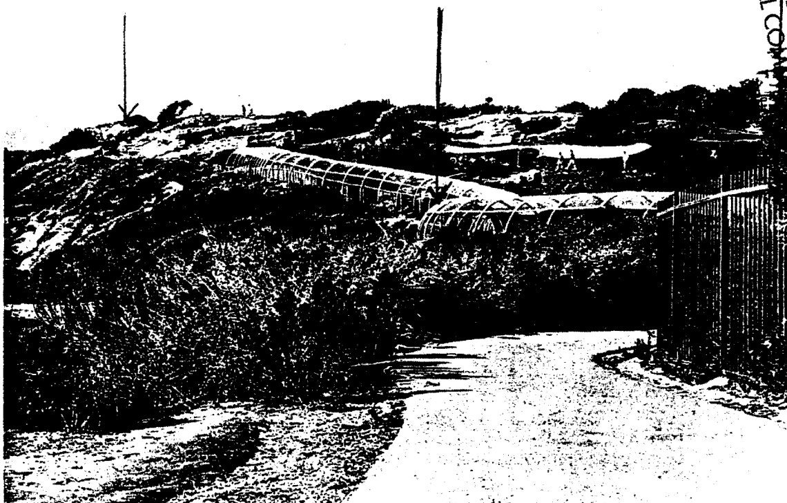
View of the existing hazard protection fence from the beach access trail. Proposed project would extend the hazard protection fence to the location of the red arrow. (150' LF) Photo also shows a close up of the type of tubular steel fence which this project will replace.
