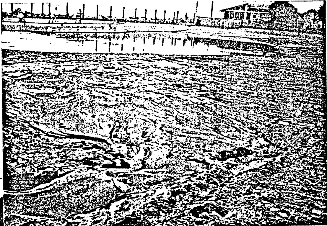
Above: Sand boils formed in Redondo Beach Seaside Lagoon beach area from liquefaction
