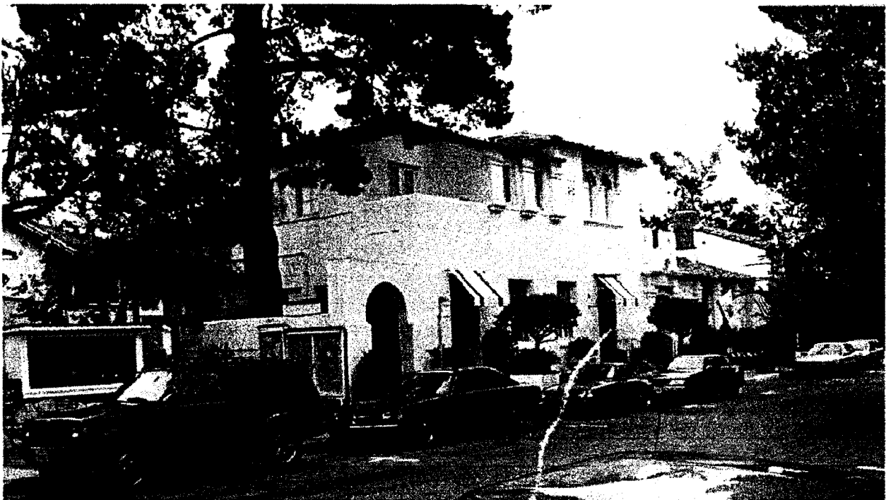
Photo 2. View of Cypress Inn adjacent to Morgan Studio site. Pine behind arched gate will be preserved in new design.
