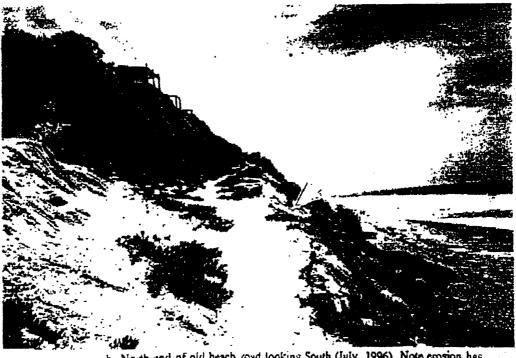
b. North end of old beach road looking South (July, 1996). Note erosion has removed much of paved portion of road in center of photo (arrow).
