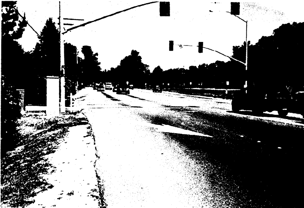
Photo 1. Highway 1 at Ocean Avenue - view looking north.
