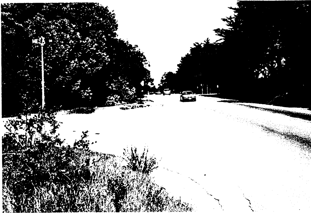
Photo 7. Southbound Highway 1 at Mesa Drive - view looking north.
