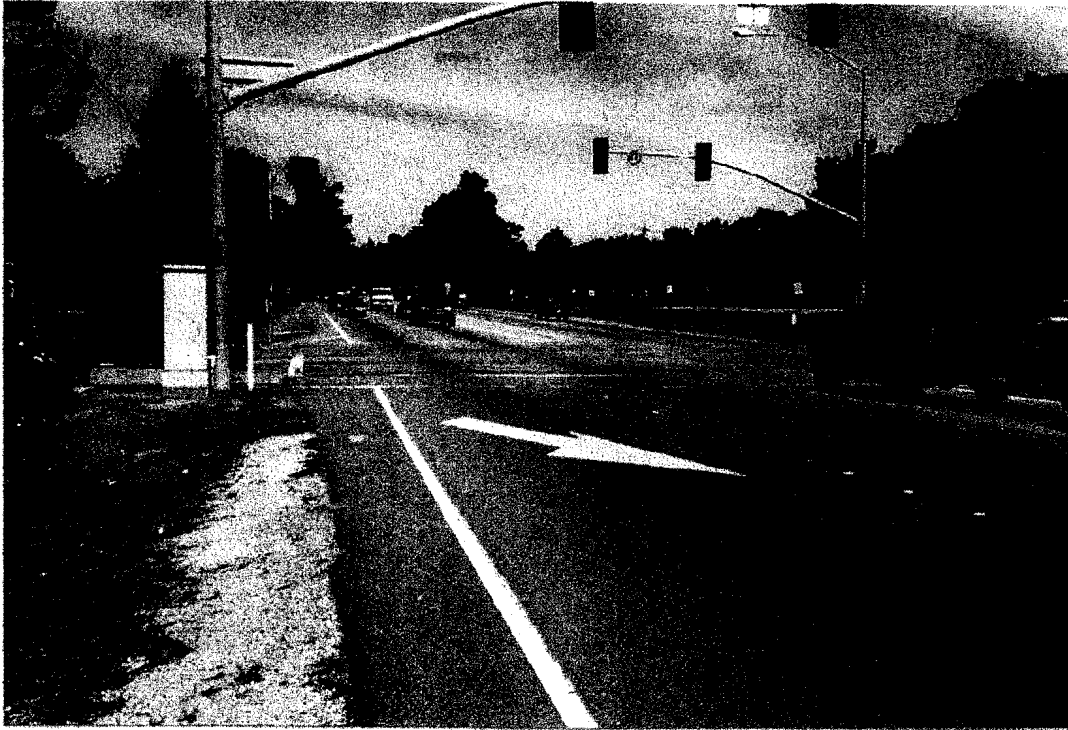
Photo 1. Highway 1 at Ocean Avenue - view looking north.
