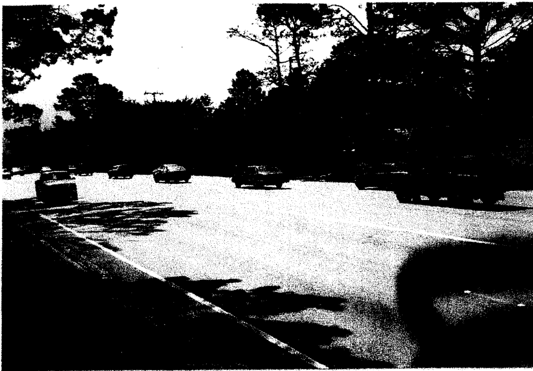
Photo 4. Wide angle view of existing merge lane Highway 1 south of Ocean Avenue - view looking south.
