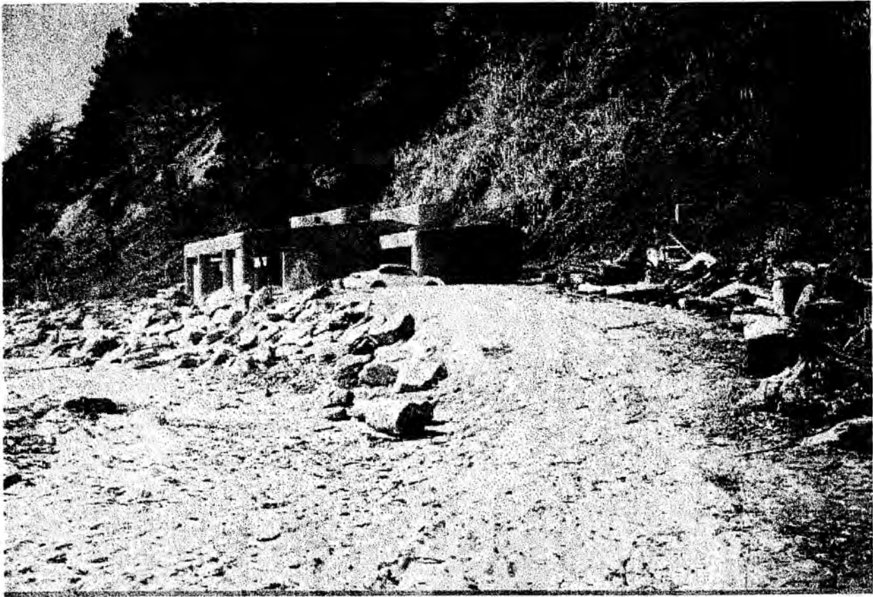
2. Looking West toward New Brighton Pump Station
