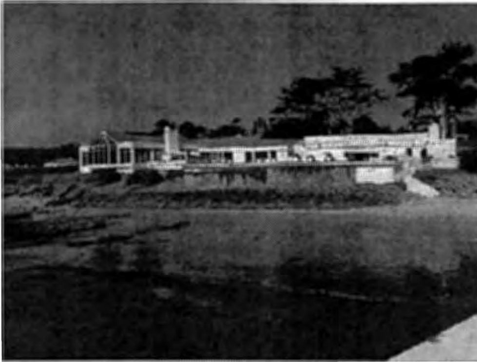
Photo 1. View of Beach Club from Stillwater Pier.
