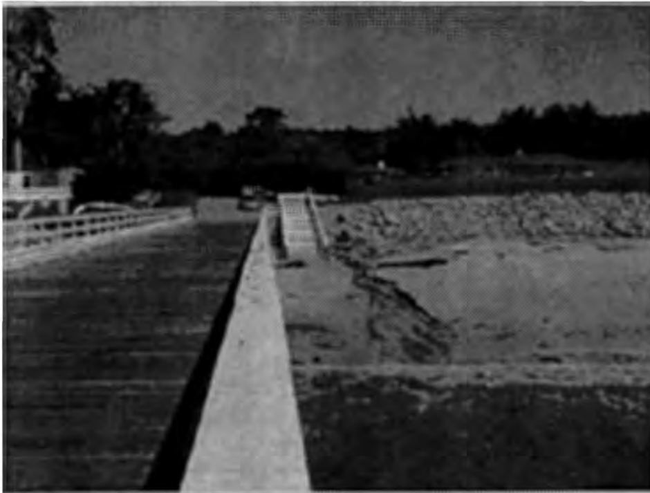
Photo 4. View of Stillwater Pier and beach access stairway from Stillwater Pier.
