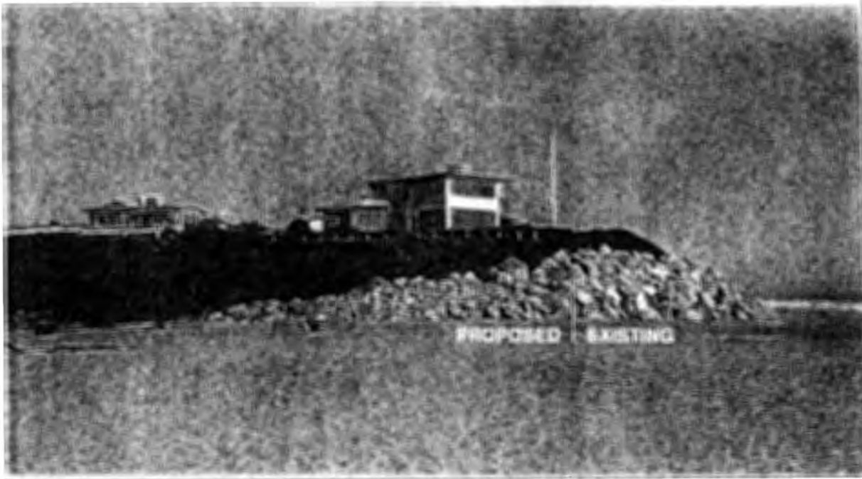
View of revetment from beach/seasonal lagoon area. Fillizetti residence is in center. Existing pathway is located below house, above rock rip-rap.
