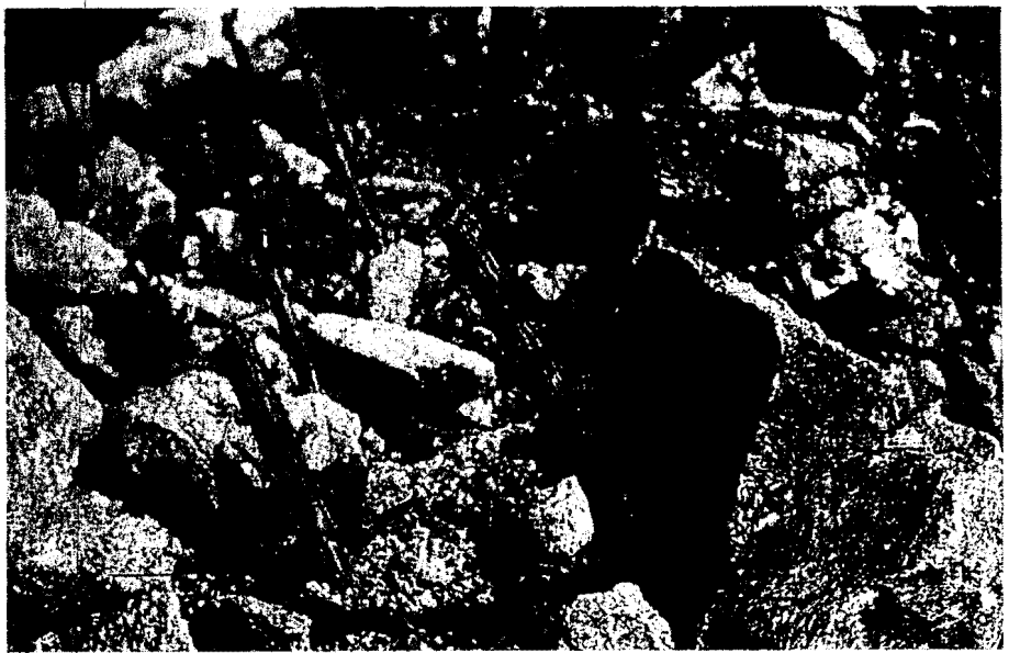
Figure 8-2. Photo of vegetated riprap revetment showing cuttings that have rooted and sprouted between the armor rocks.
