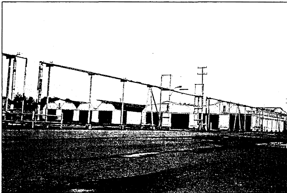
PHOTO #12 (P12) Dry kilns to be removed. Elevated steam line is shown through middle of photo.
